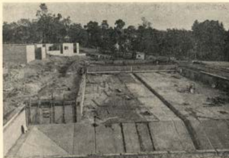
MAIN POOL UNDER CONSTRUCTION
