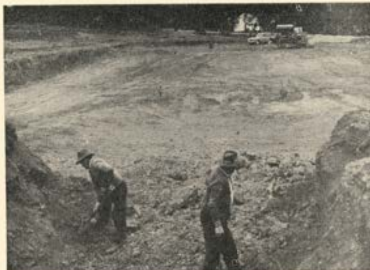
EXCAVATING THE SITE
