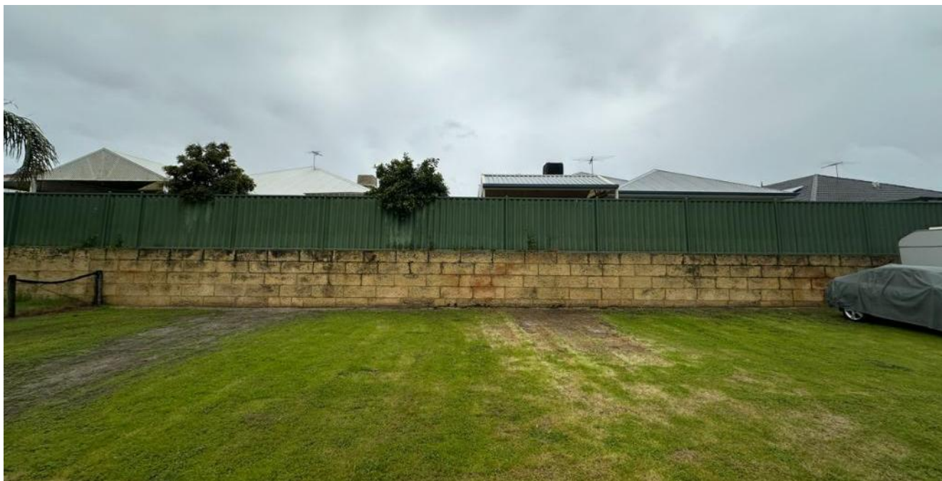
Photograph 8: Near BH15 facing south east
