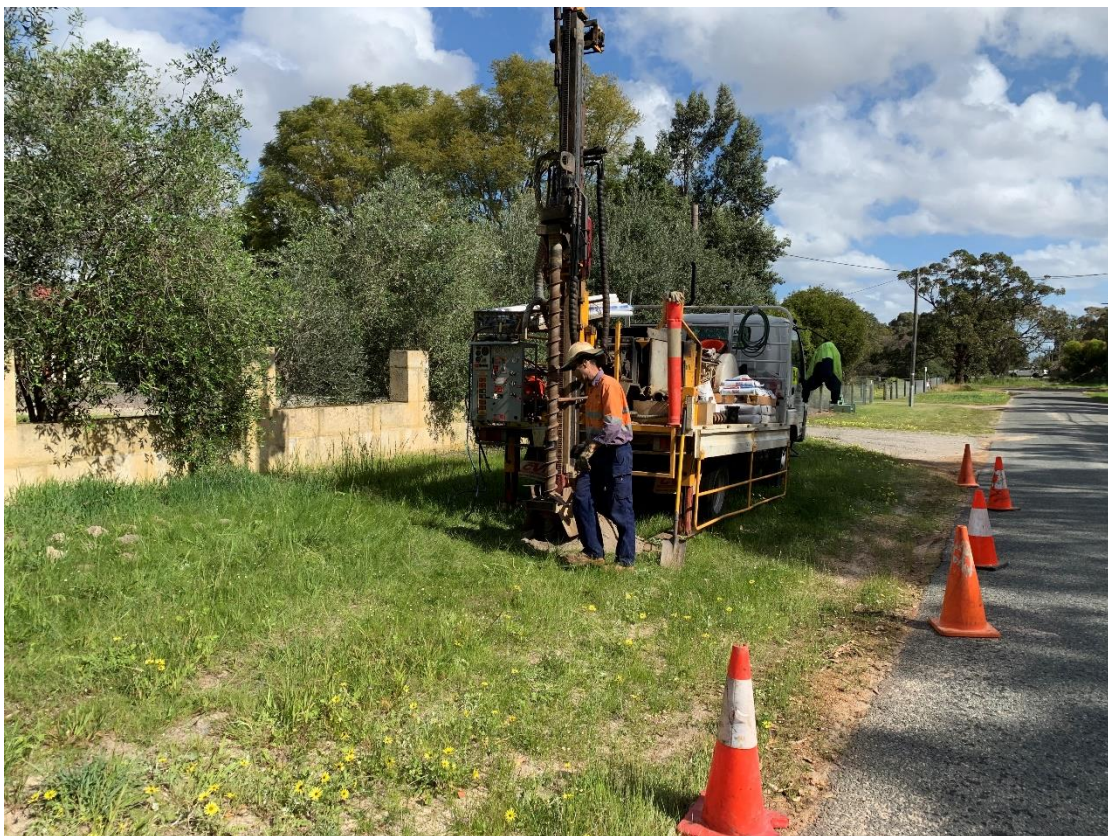
Figure 2: Drill rig on location
