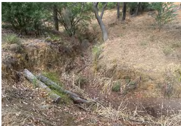
Plate 2-6: Eastern embankment of Crystal Brook
