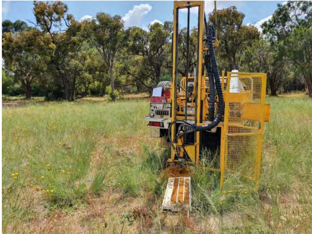
Photograph 3: Borehole drilling at the north of the site
