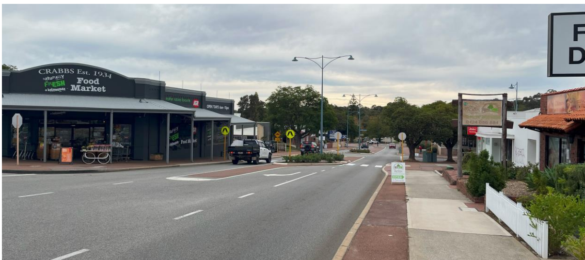
Photograph 2: Existing IGA supermarket and Canning Road streetscape to the north
