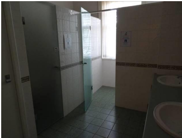
Figure 76 Bath 1 (former dressing room)
