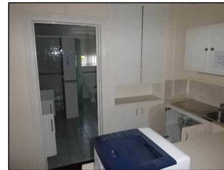
Bathroom 3 – Kitchen bench may obstruct ease of access if this bathroom is repurposed as a unisex accessible toilet
