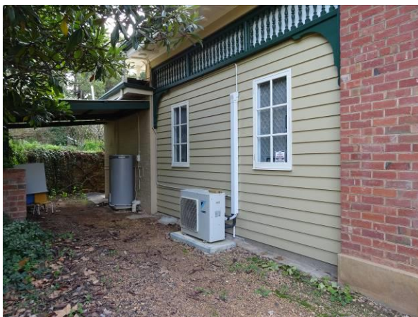
Figure 44 South elevation, showing lean-to to be demolished
