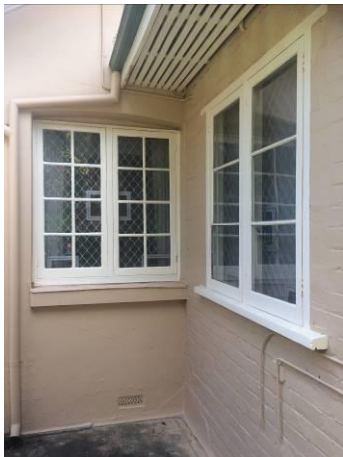
Figure 42 View of windows to bathroom 2 & bedroom 4
