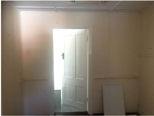
Figure 113 Bed 6, north wall
