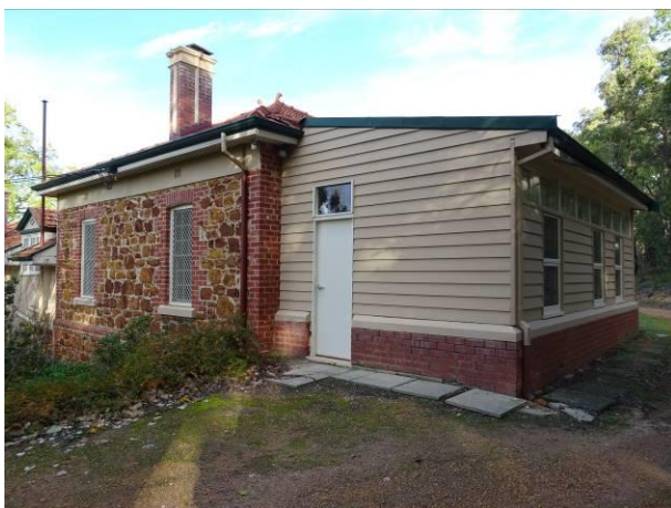
Figure 22 North facade, sunroom
