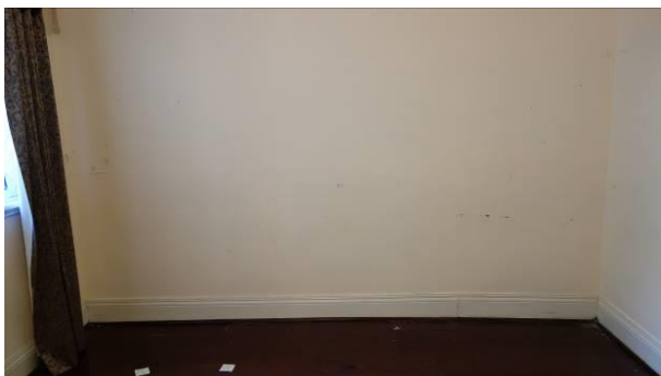
Figure 85 west wall, bed 4
