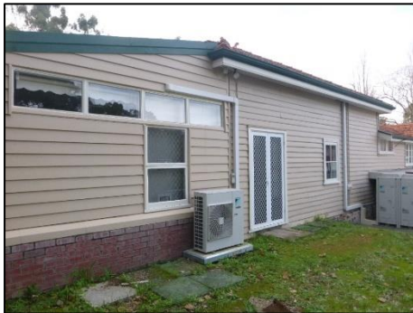
Side door that may form a new, principal entrance to the Upper Level
