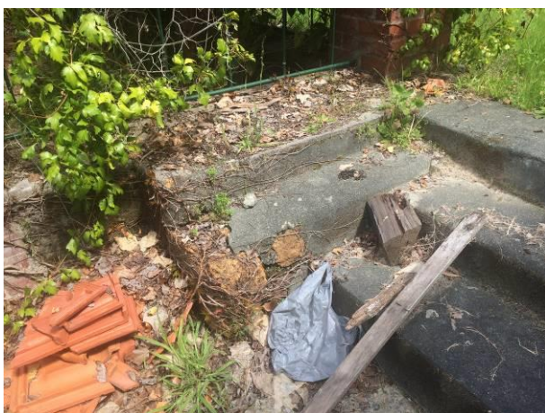
Figure 32 Stairs to condenser unit area
