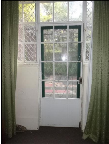
Bedroom 3 with metal framed door and matching adjacent windows
