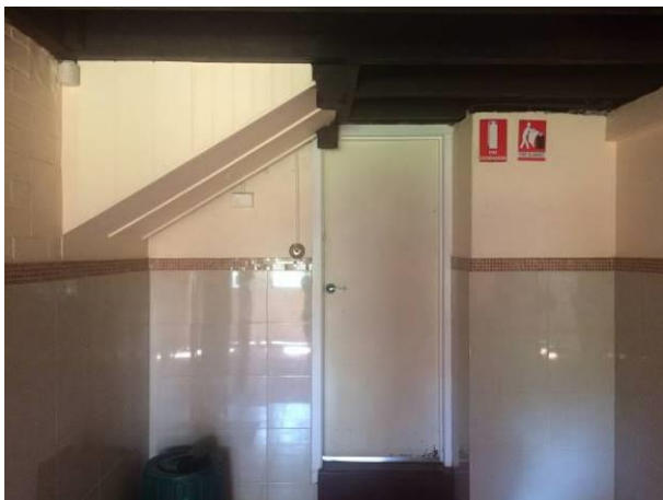
Figure 105 Mudroom, south wall
