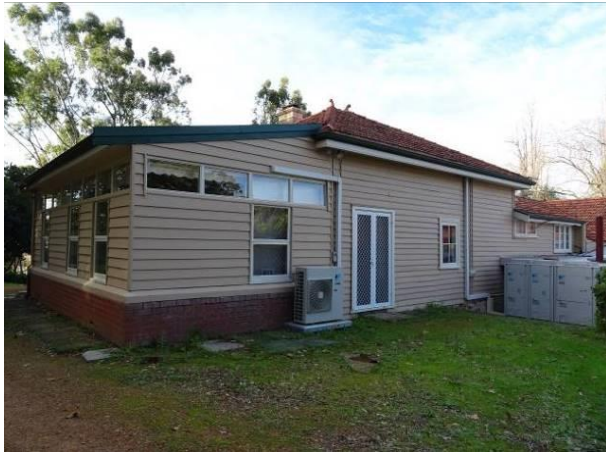
Figure 29 South facade of Upper Level
