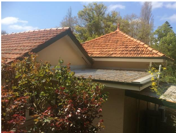
Figure 36 West facade, roof over bathroom 2
