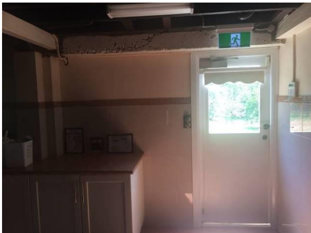
Figure 103 Mudroom, north wall
