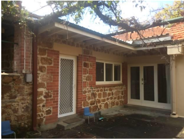
Figure 40 View of Kitchen and Dining room doors
