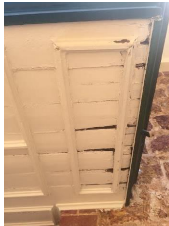
Figure 16 Soffit of main entrance canopy
