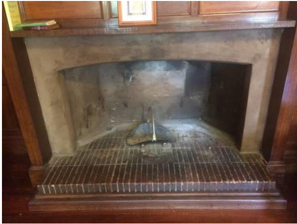
Figure 69 Panelled room fire place
