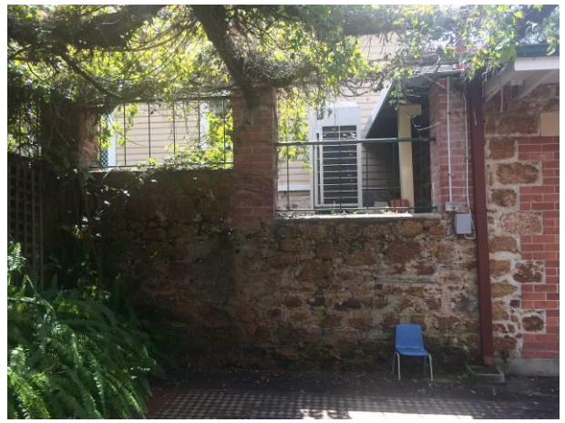
Figure 39 Courtyard wall looking north
