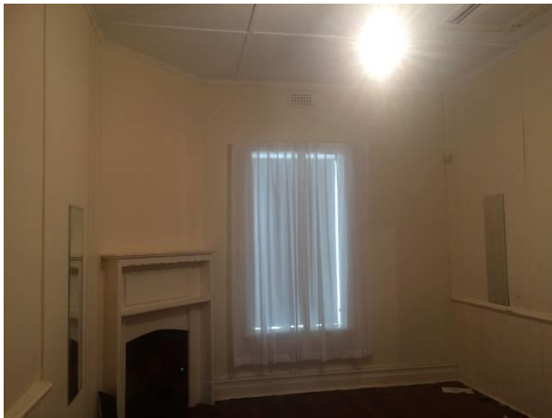
Figure 117 Bed 7, north wall
