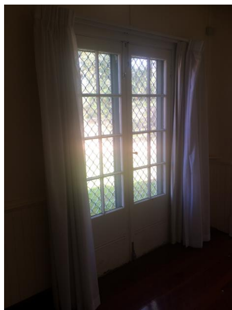
Figure 112 external doors, upper hall
