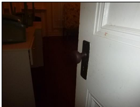
A knob style handle is non-compliant. Further consultation may be necessary if these are deemed an essential heritage element to be retained.
