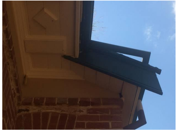
Figure 14 Exposed downpipe in gutter
