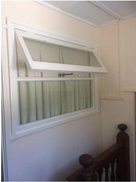
Figure 107 Stair landing, upper floor
