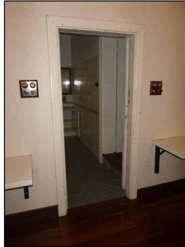
Bathroom 2 door with Bedroom 4 door in the background (with steps)
