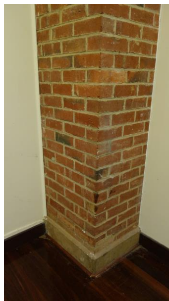
Figure 92 Bed 5, brick pier
