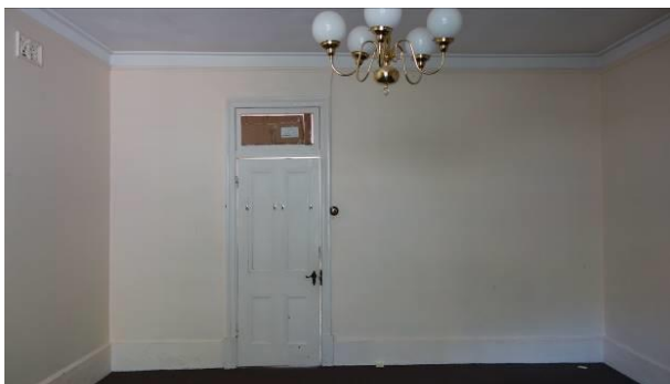
Figure 81 east wall, bed 3 (original dining room)
