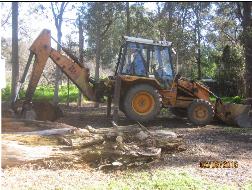
Photo 7. Test Pit location 03 (TP3), sub-surface probing by using backhoe
