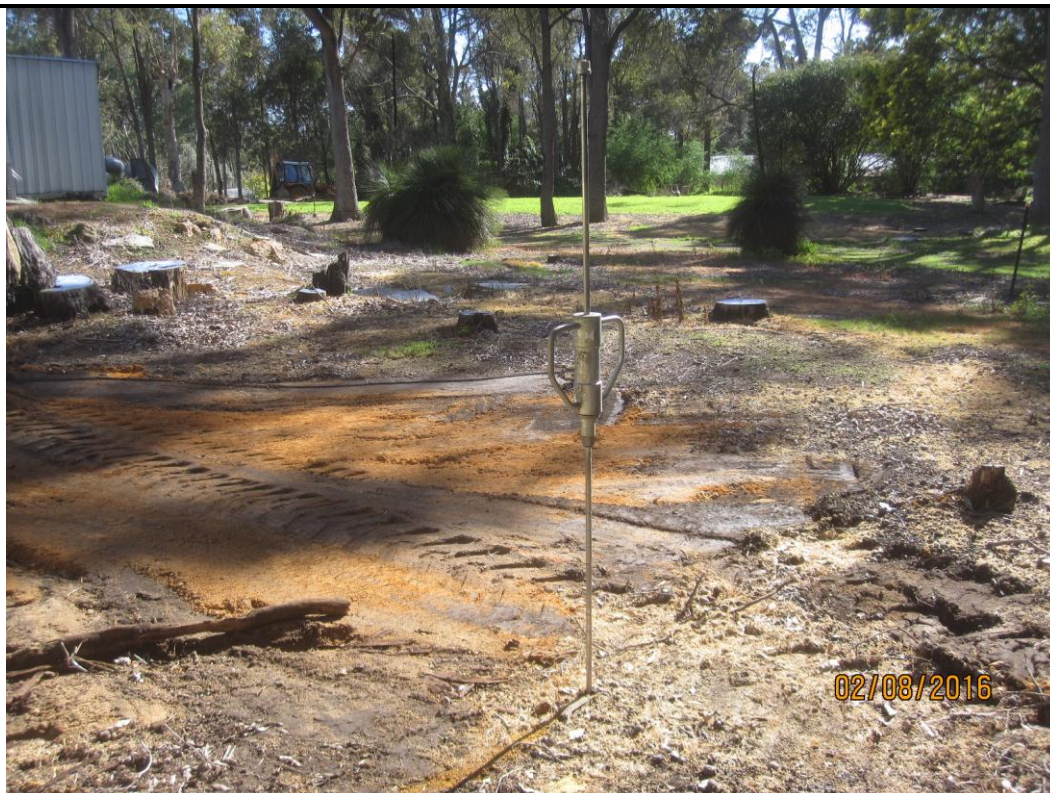
Photo 9. Test Location DCP2, Conducting Dynamic Cone Penetrometer Test
