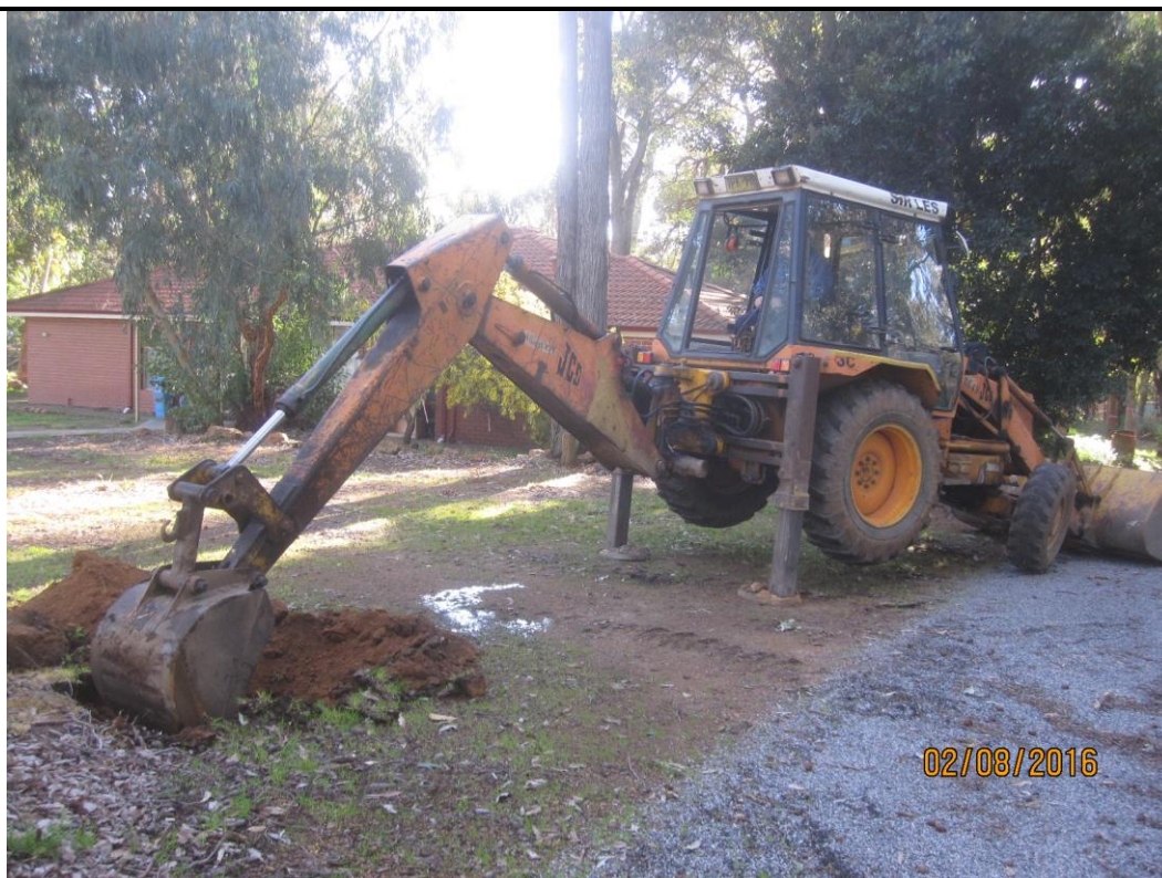
Photo 4. Test Pit location 01 (TP1), sub-surface probing by using backhoe
