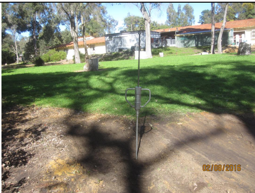
Photo 10. Test Location DCP4, Conducting Dynamic Cone Penetrometer Test
