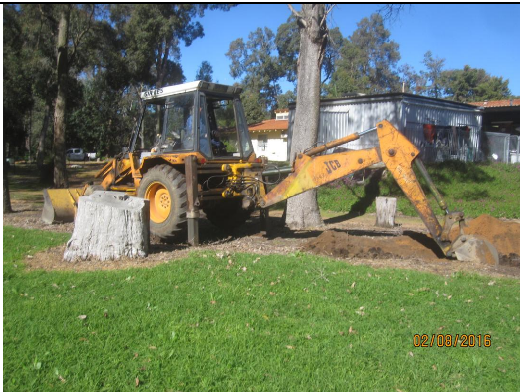
Photo 8. Test Pit location 06 (TP6), sub-surface probing by using backhoe
