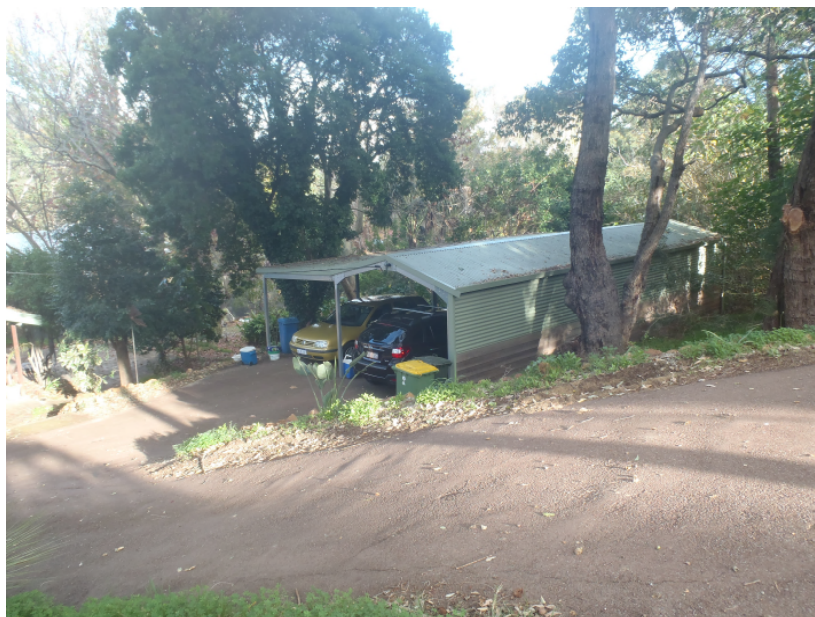
Photo 4: Staff parking at 59 Coolinga Road
