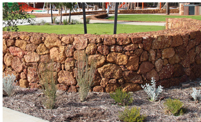
LATERITE STONE WALL
