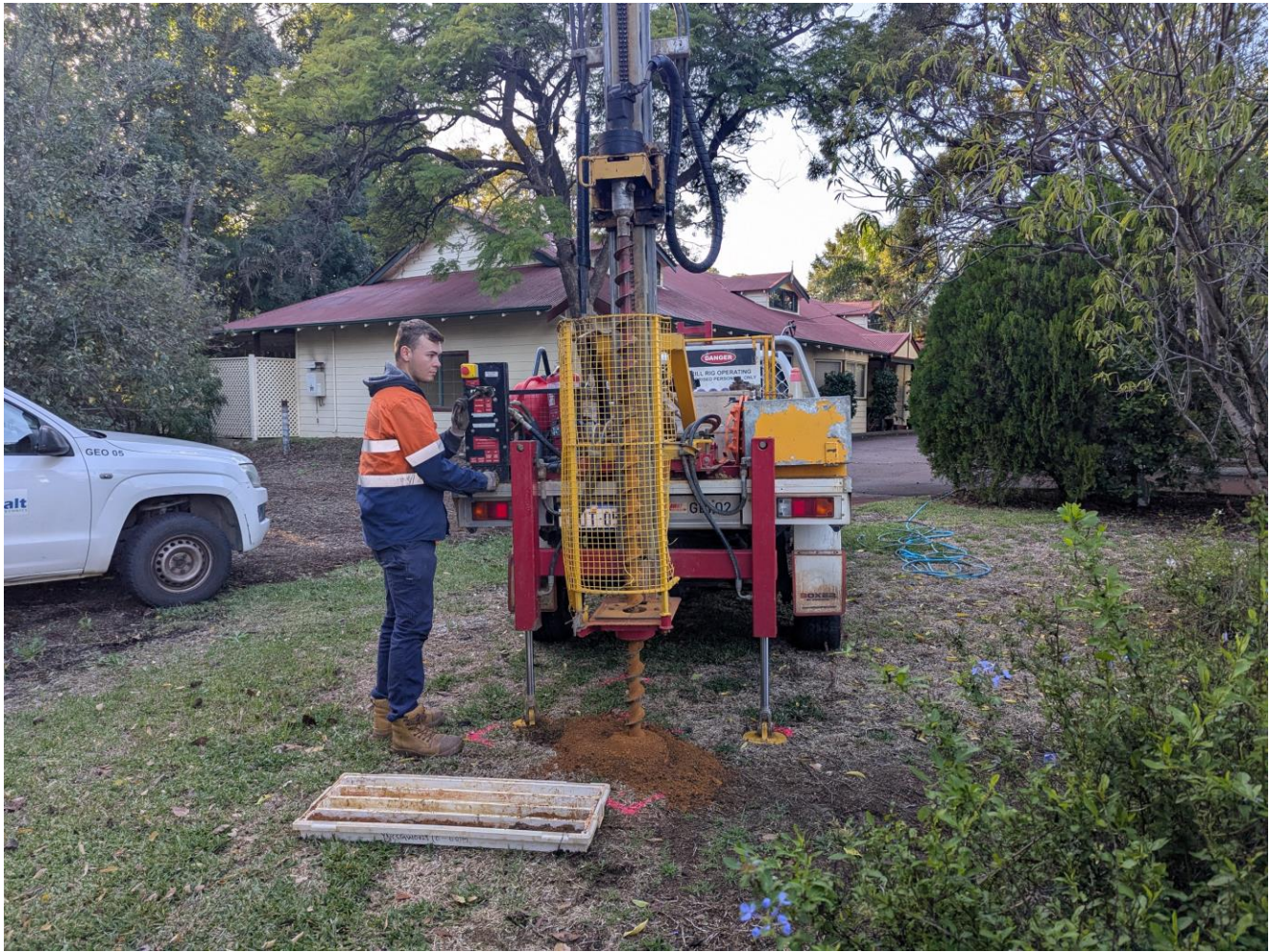
Photograph 2: Borehole drilling underway
