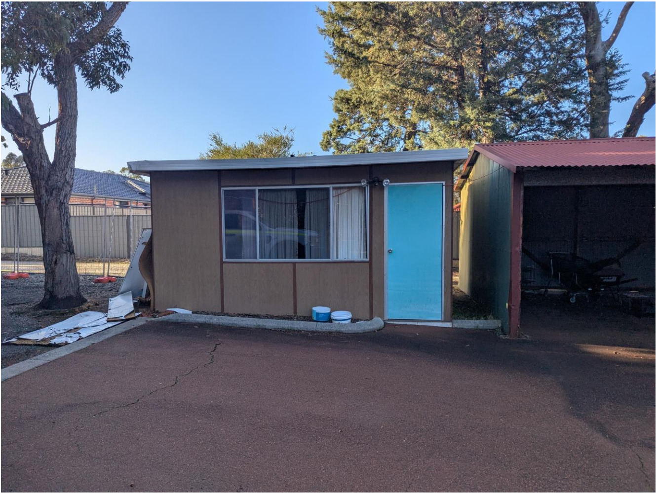
Photograph 4: Looking at existing asphalt pavement and outbuildings.
