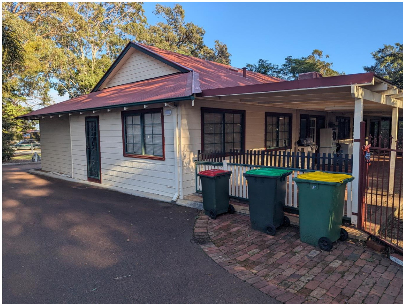
Photograph 3: Looking at existing building at the site.
